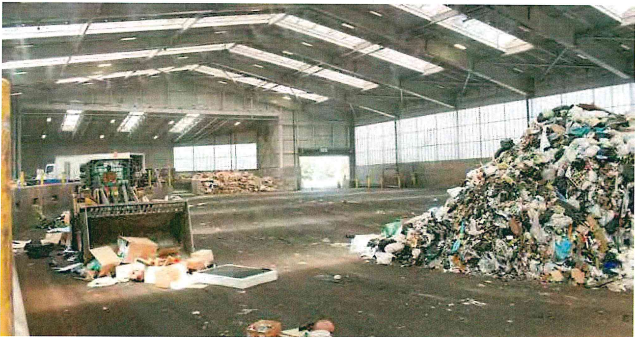
Bow Lake Recycling and Transfer Station
