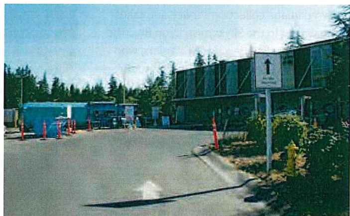
The Vashon Recycling and Transfer Station
