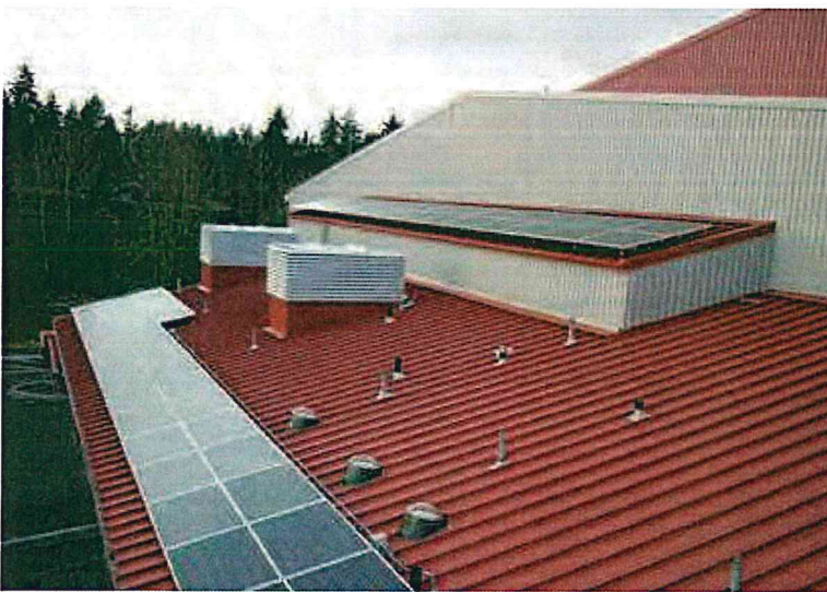
Solar panels on the south roof of the Shoreline Recycling and Transfer Station, one of the many green features of the building
